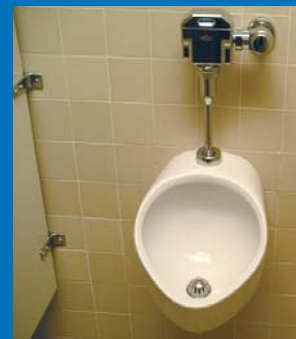
The Zurn Nano Pint urinal uses just 16 ounces of water, is designed for retrofit applications, and saves up to 96% in water usage compared to 3.5 GPF fixtures.
